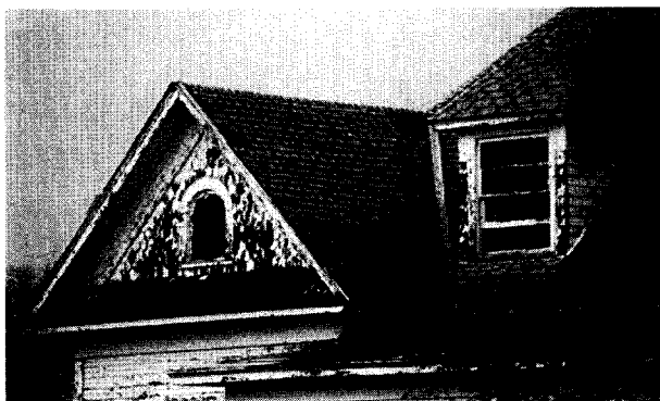
Above: Hail damaged the siding and broke windows of this house along U.S. Highway 581, west of Lometa. Above(right): A volunteer fire station in Lometa with north facing bays was damaged by the wind.
